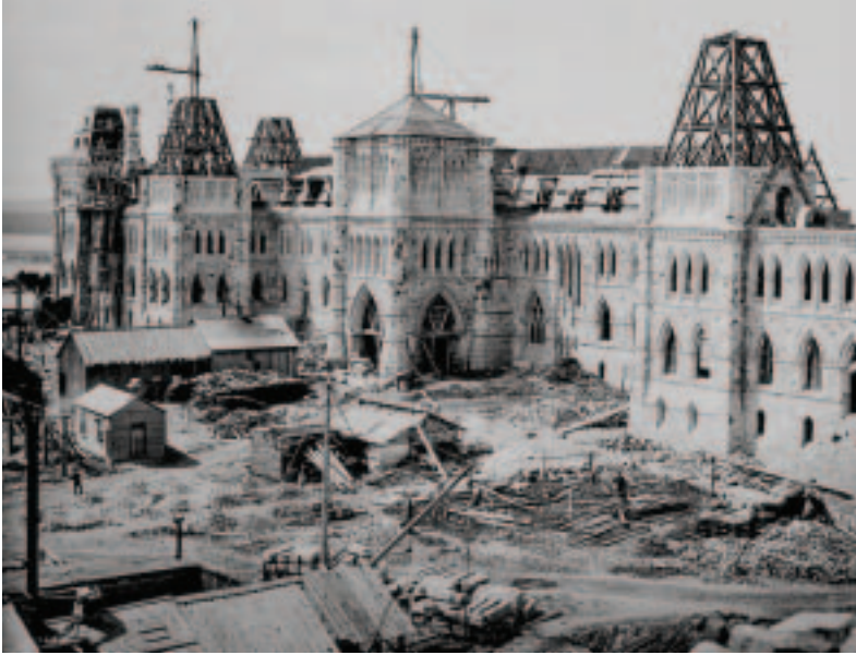
Parliament building under construction in 1863
